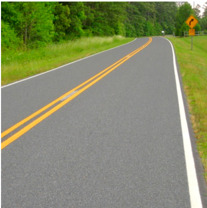
Typical \frac{5}{16} " Asphalt Surface Treatment seal
