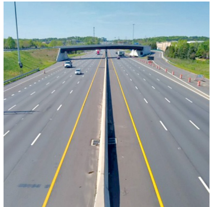
Stalite Lightweight Aggregate hot mix on I-85
